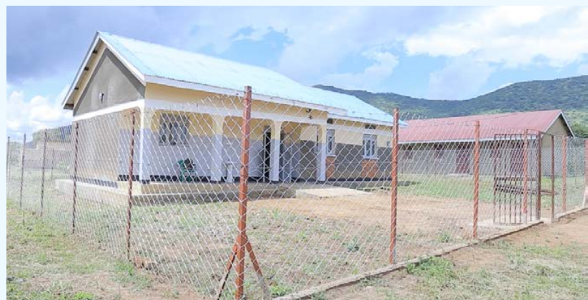
A fully stocked honey processing centre renovated and equipped under BAC1 with funding from word en Daad.
